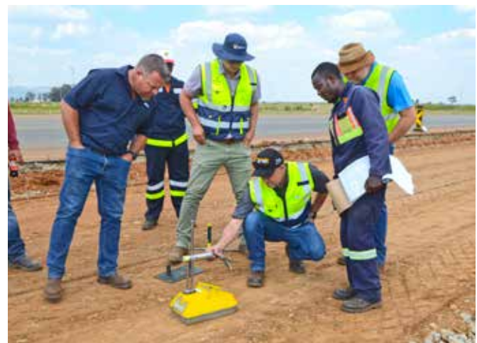
JCB compaction specialists at a JCB Roller Day in Johannesburg.
