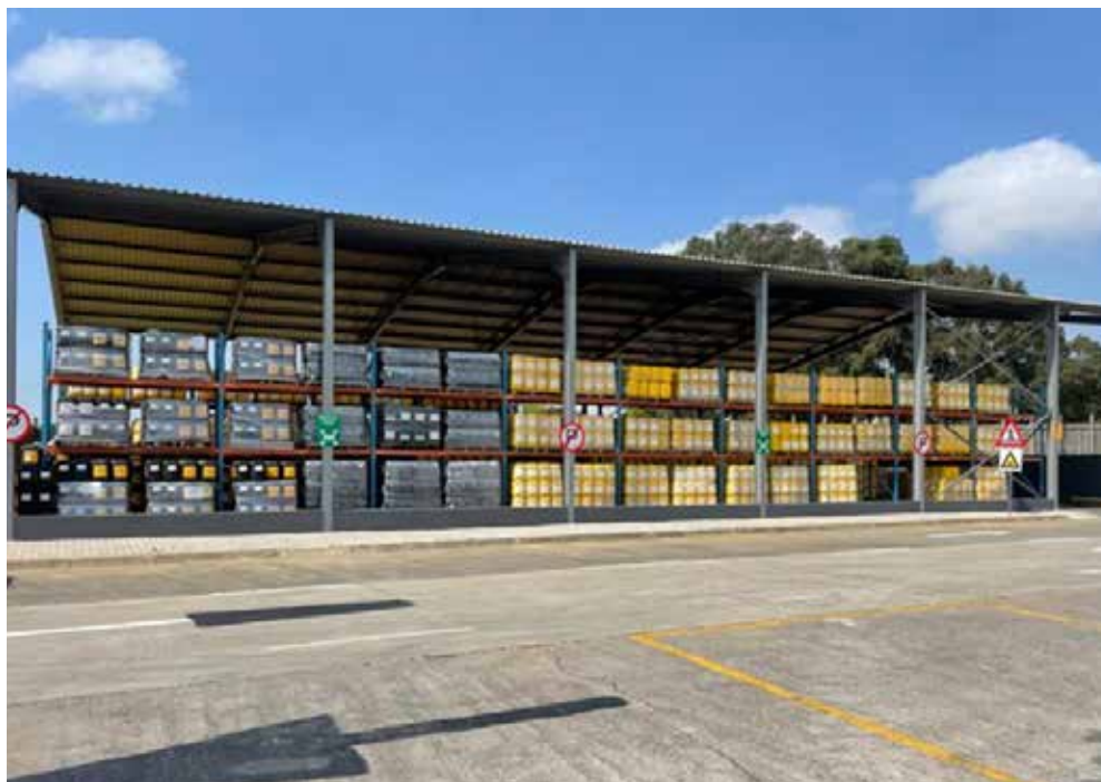
A new bulk oil storage facility was constructed at the GLC, which complies to the latest environmental requirements pertaining to hydrocarbon storage and will ensure minimal risk in terms of hydrocarbon contamination into the storm water system.
